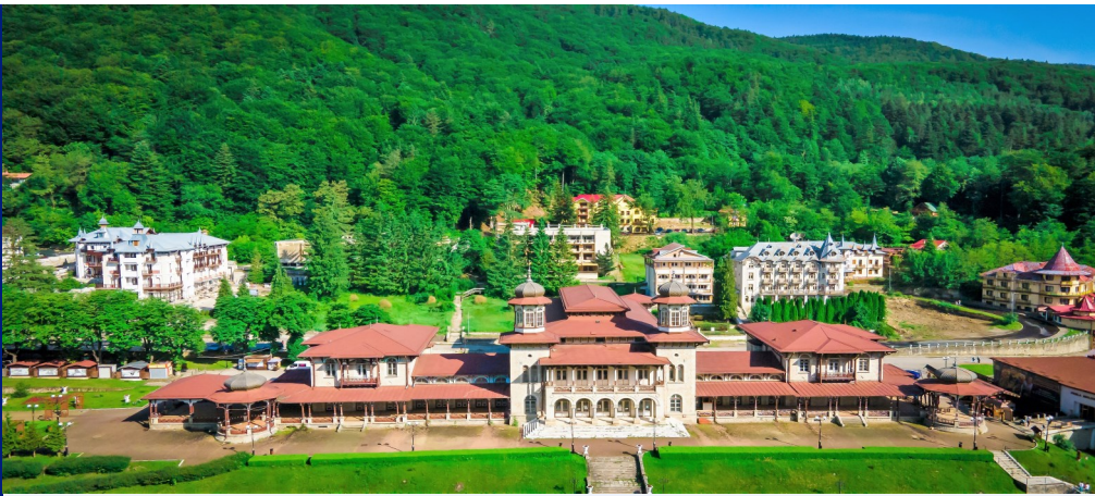
Slănic-Moldova has a high-performance SmartArt City type air quality monitoring system.
